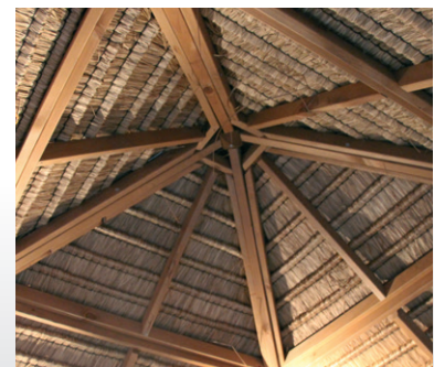
PRE-FABRICATED THATCH ROOF
